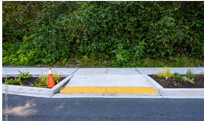
Planted structural curb extensions can enhance the streetscape and capture street run-off while slowing traffic.
