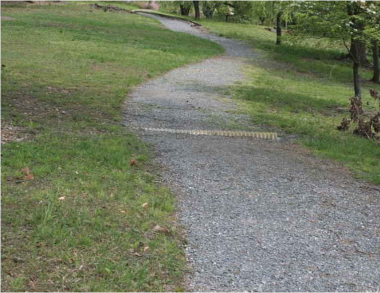
Trail surface erosion exposes a corrugated metal drain pipe.
