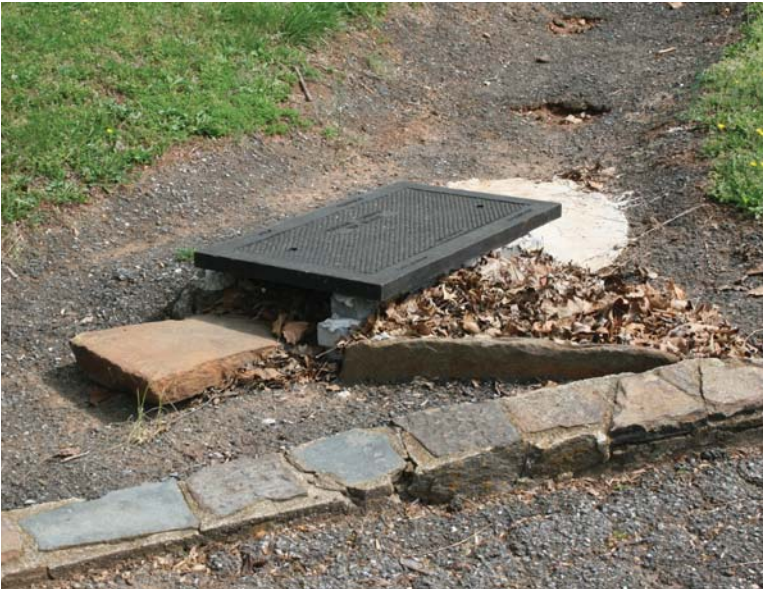
This drainage structure is blocked and water flow is prohibited.
