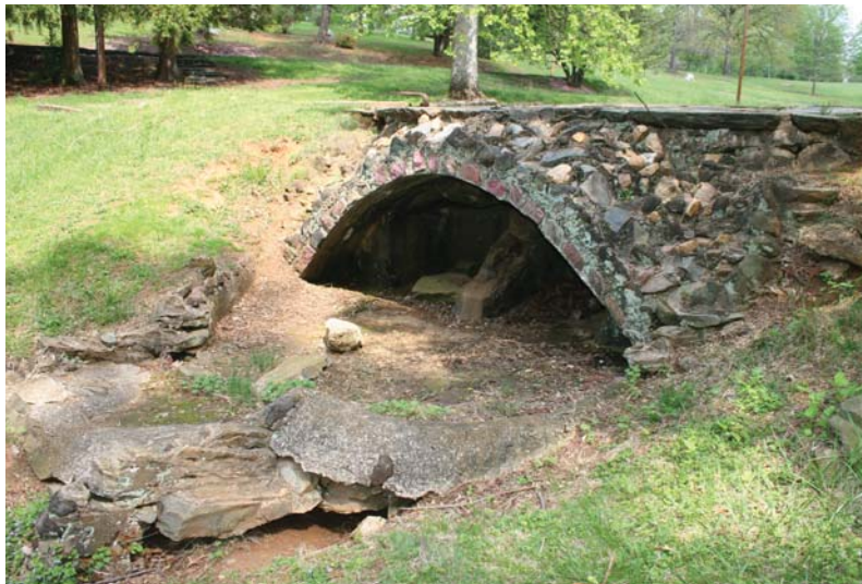
Remnant of the pool drainage structure that channeled water to the Old-Fashioned Garden.
