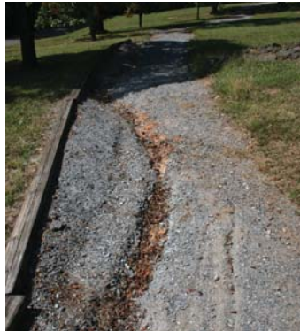
Erosion damage on gravel trail.
