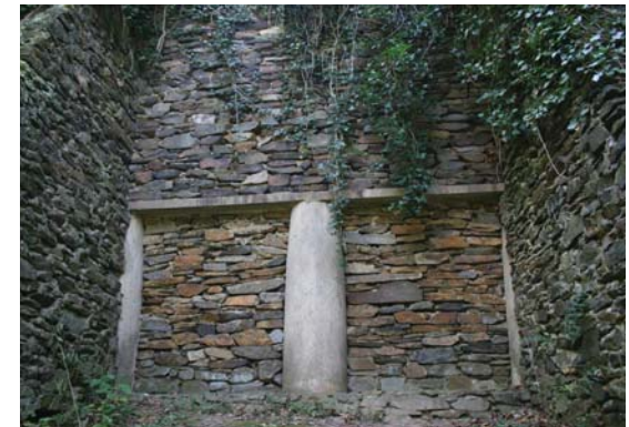
Salvaged buttresses supporting the stone overlook.
