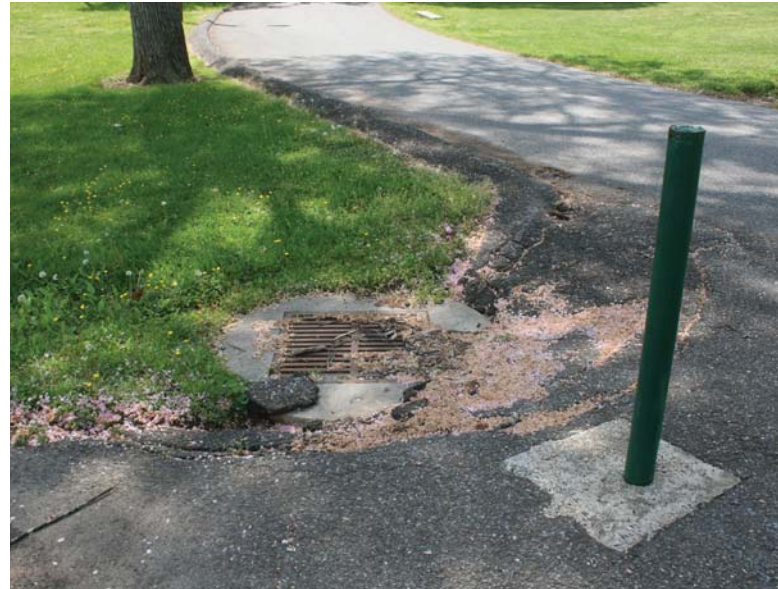
This drainage structure is damaged due to pavement disintegration.
