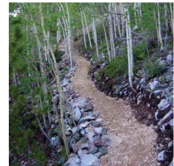
Where the trail follows the bluffs it may need to be stabilized. Riprap is one option, as shown.
