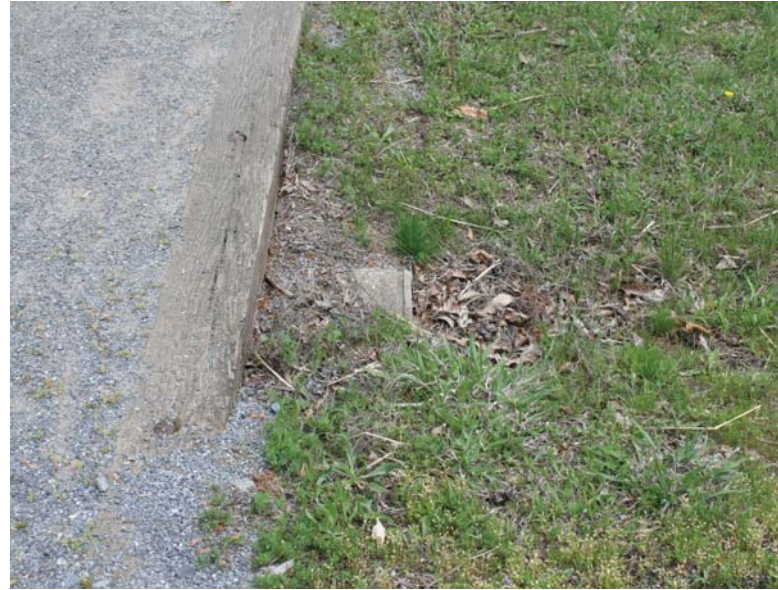
Leaves and soil fill a drainage pipe that passes under a trail.
